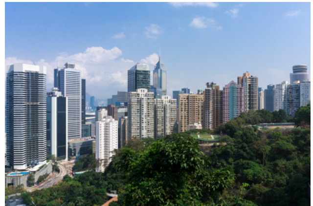
At the end of March, AHK Greater China hosted a digital business delegation in Hong Kong for German SMEs active in the building energy efficiency market
